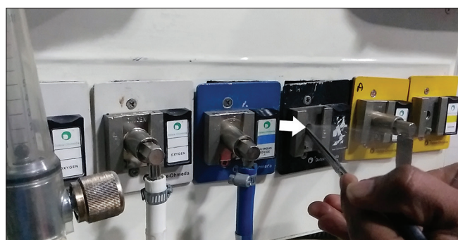
Figure 2: Water being purged from central supply system (arrow)
